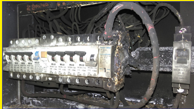
Make sure you get your switchboard and electrical equipment checked for safety before it's too late.
